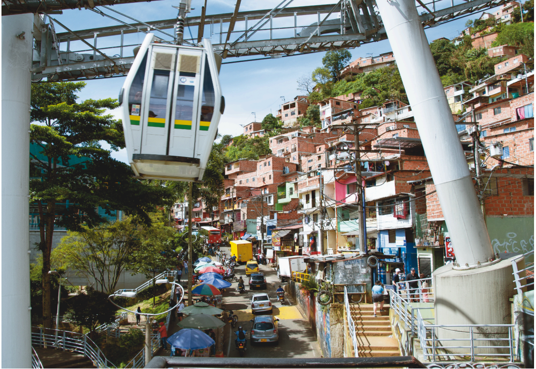
Figure 4: A cable car passing by the barrio of Santo Domingo.
