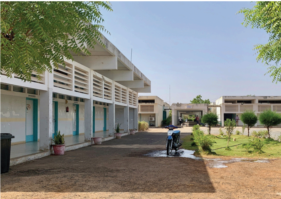
Figure 3a: Heinrich Lübke Regional Hospital in Diourbel, Senegal, architect: Lippsmeier + Partner. State: May 2022.
