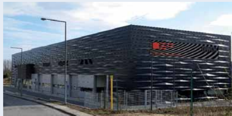
Versuchshalle E.ON Energy Research Center, RWTH Aachen
