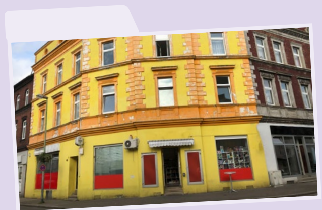
Problemimmobilie in Essen
