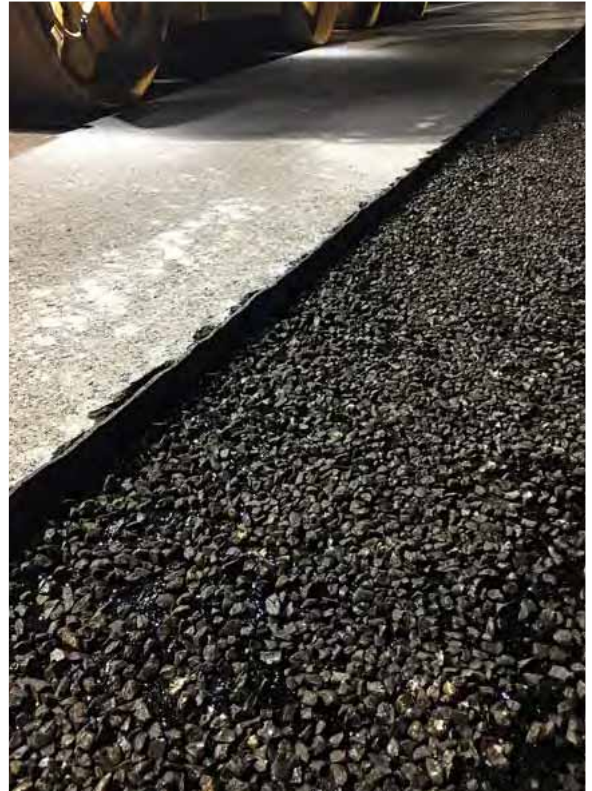
Applikation der SAMI (Stress Absorbing Membrane Interlayer)
