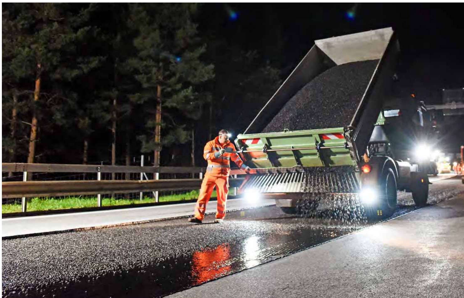
Applikation der SAMI (Stress Absorbing Membrane Interlayer)
