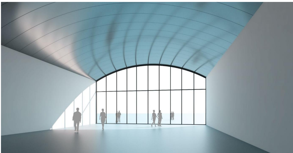
Abbildung 4-3: Hallen Dach aus einachsig gekrümmte Elementen Figure 4-3: Roof made of single curved elements
