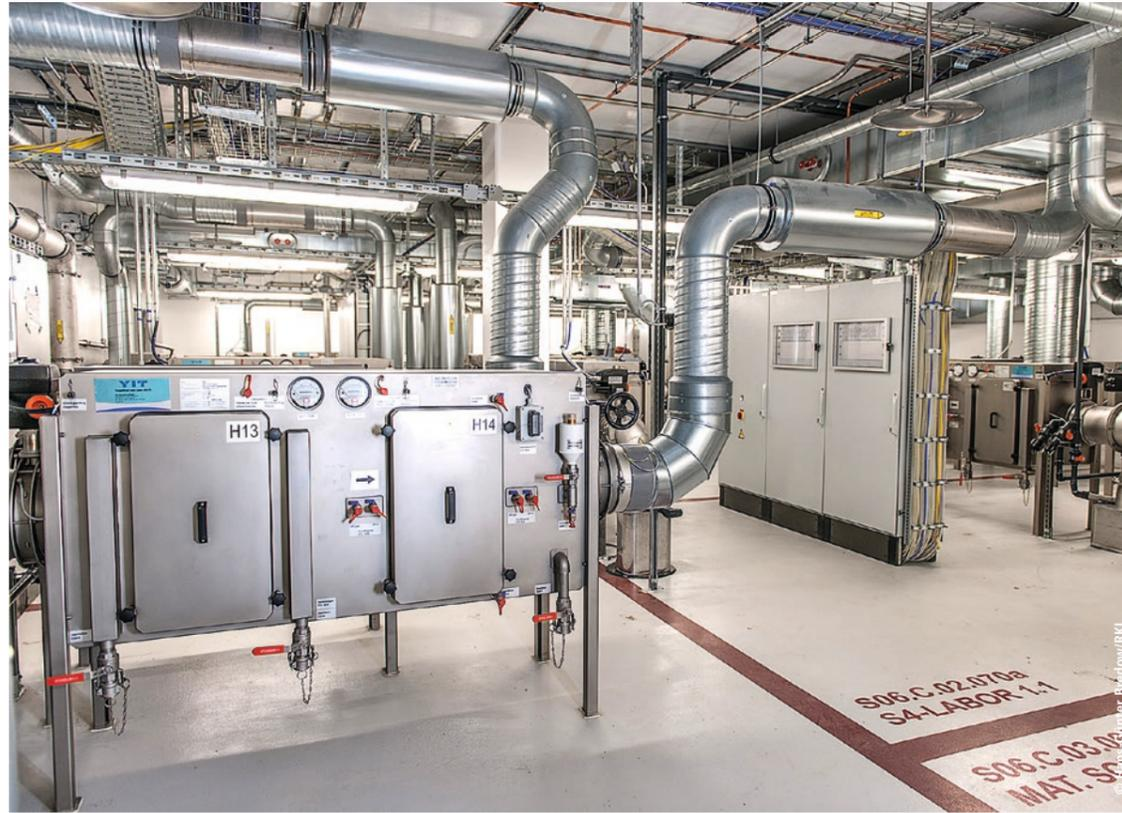
To ensure no pathogens escape, all outgoing air from the high security laboratory is treated with a multi-level filter system with highly efficient filters (HEPA filters). The outgoing air flow rate is more than 20,000 m<sup>3</sup> per hour.
