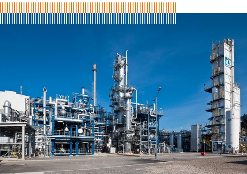
Air Liquide hydrogen production site
