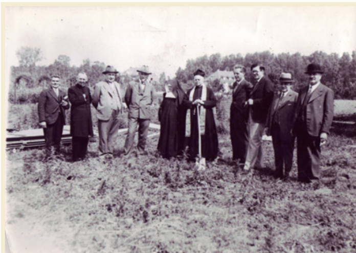
Spatenstich KKH St. Elisabeth © Archiv KKH
