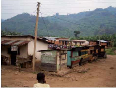
Electricity Grid at Nyamyotsi [NIC]
