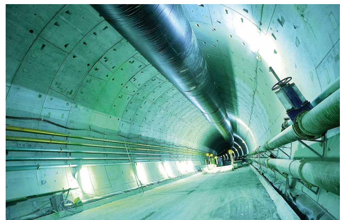
Sealed tunnel made of tubing segments
