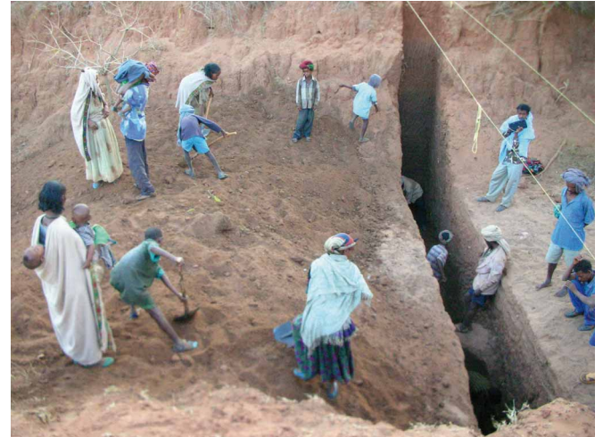
Construction of the first groundwater dam in Koraro (Tigray). MUAS (2)
