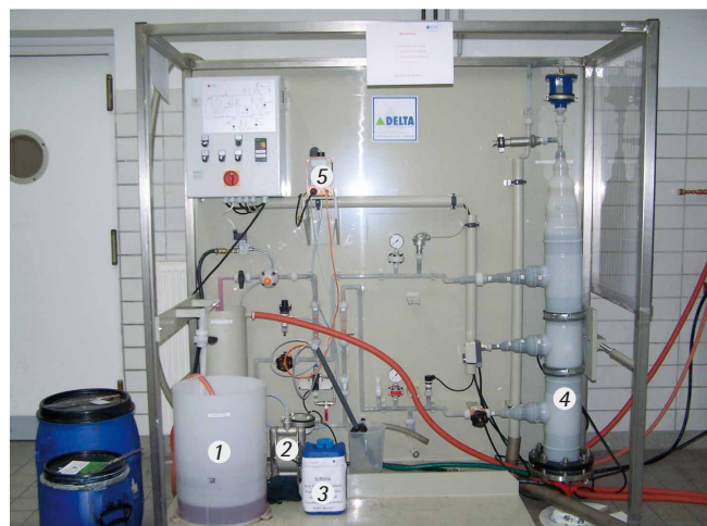
1: Coloured wastewater, 2: Circulation pump 3: H 2 O 2 reservoir, 4: Oxidation reactor, 5: Dosing pump for H 2 O 2
