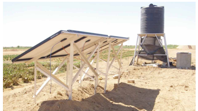
Solar powered low pressure irrigation system at the trial station of the OWARA project
