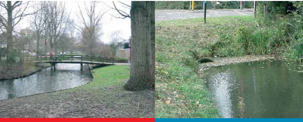
Polluted water from the sewer in a living quarter comes up to the surface.
