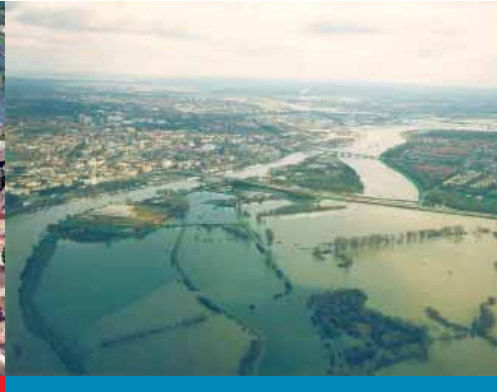
Aerial view of the pilot project site during flooding
